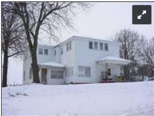
522 West Main (building to be removed by City)
